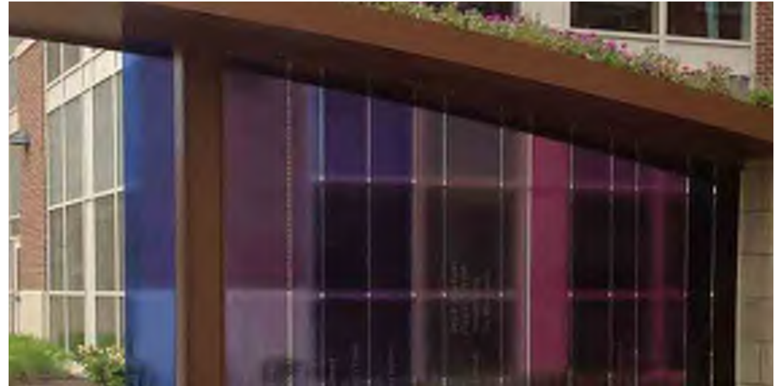
Texts printed on translucent polycarbonate panel
